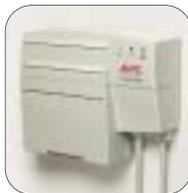
Your BBU was installed in a location in your home where it can be easily monitored. It contains a series of indicator lights that tell you whether your service is being powered by your home's electricity or the battery.
