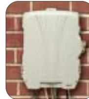
Optical Network Terminal or ONT. That way, it can be "read" by your telephone and computer. Information that is sent *from* your house will be converted from the electric signals to light in the ONT.
